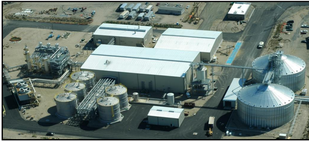
Port of Morrow—Pacific Ethanol Production Facility, 40 Million Gallons/Year ($120 million Annual Product Value)
