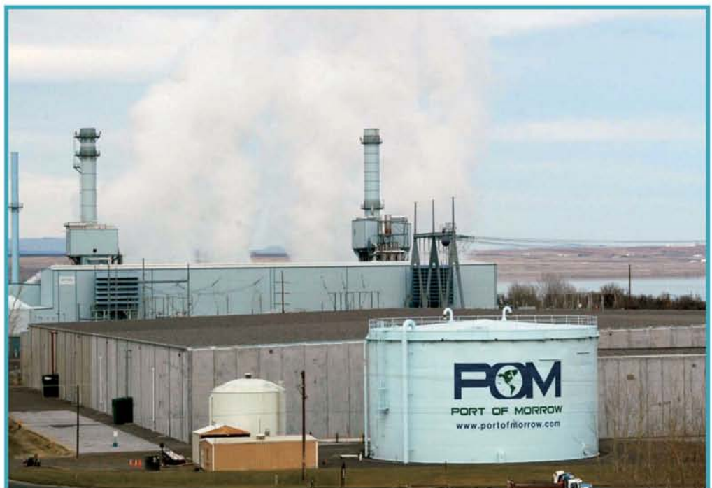
POM water tower with new paint and lettering. The building behind is the new expansion of Morrow Cold Storage.
