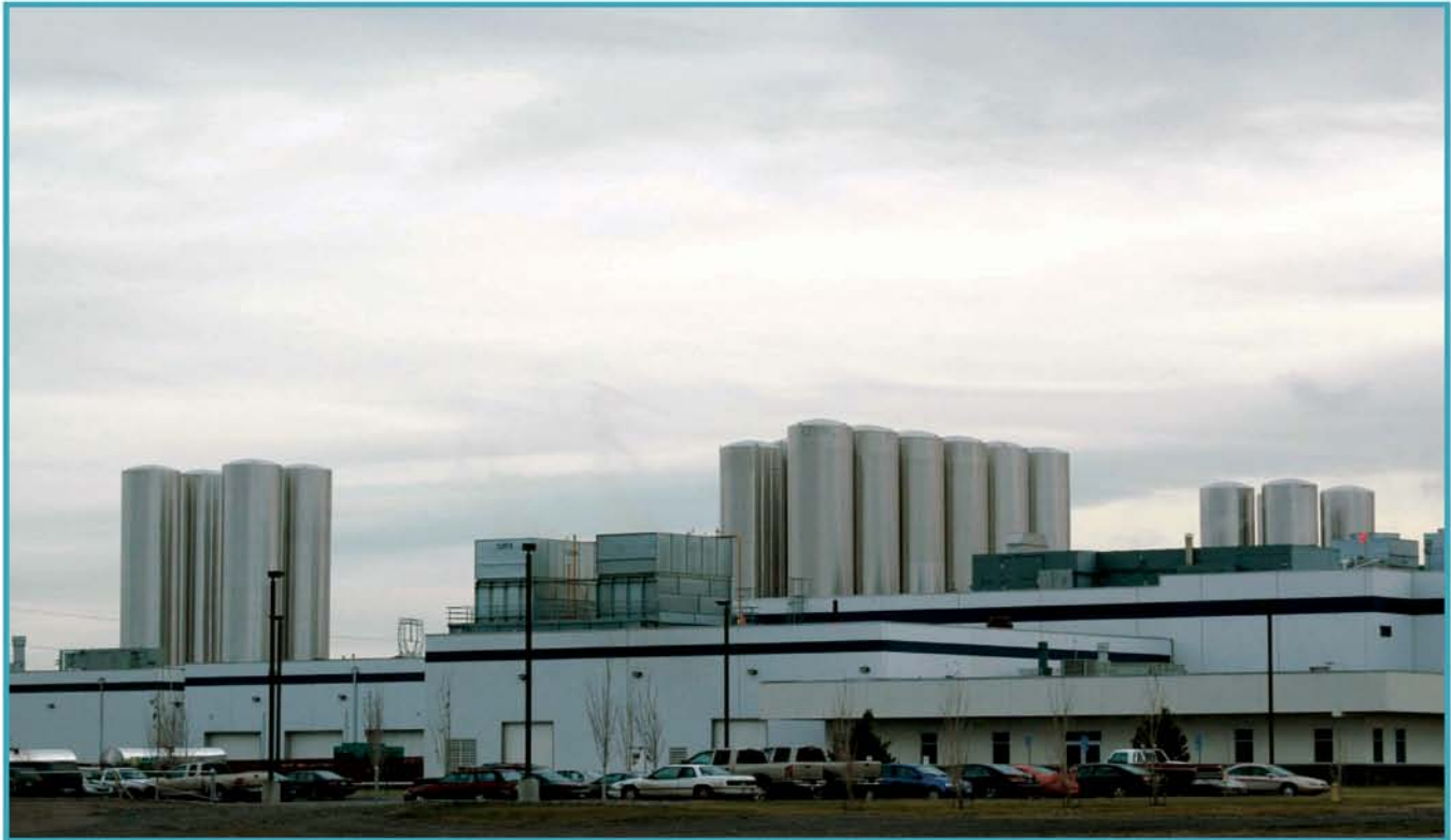
Columbia River Processing. Expansion is shown on the left.
