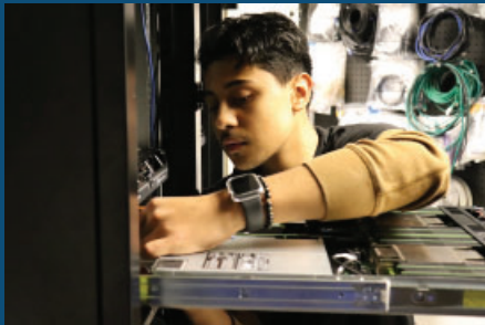
Edwin, Riverside High School Information Technology at Port of Morrow
