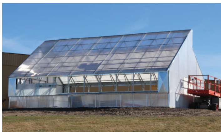
The FFA greenhouse under construction in early February
