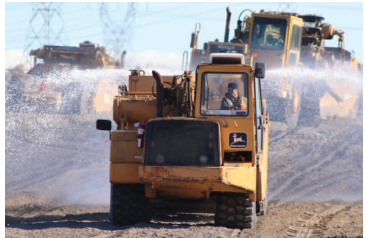
Earthmovers level ground at the flex space construction site
