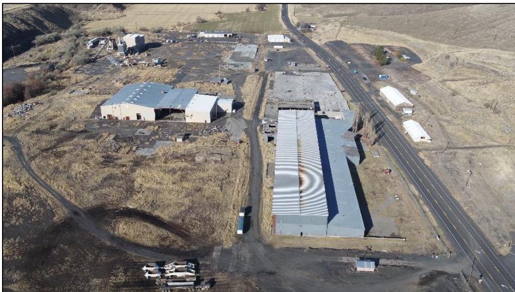
Figure 5 – Aerial of South Morrow Industrial Park
