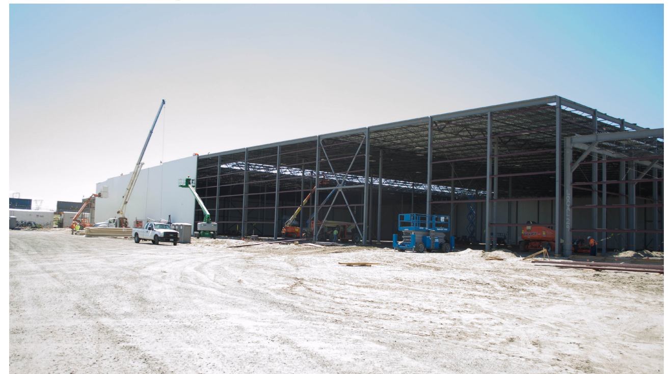
Anna Aylett photo Port of Morrow Warehousing opened June 2015 and by August of that year was full with requests for expansion. The expansion is set to be finished by October 2016 or sooner.
